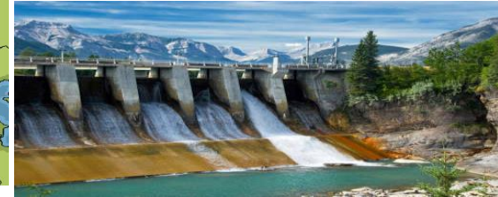
Hydropower plant in Norway.
