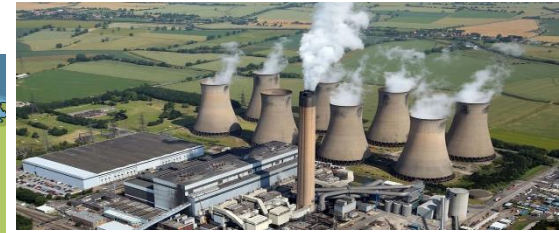
Power station in the UK.
